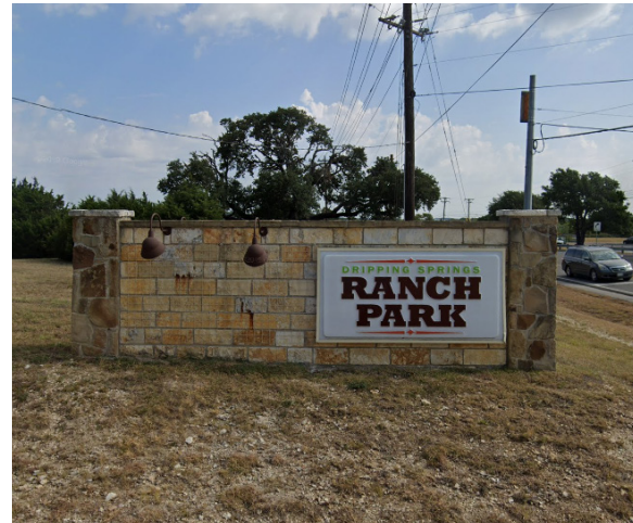
RANCH PARK ENTRANCE MONUMENT SIGN (TO REMAIN)
